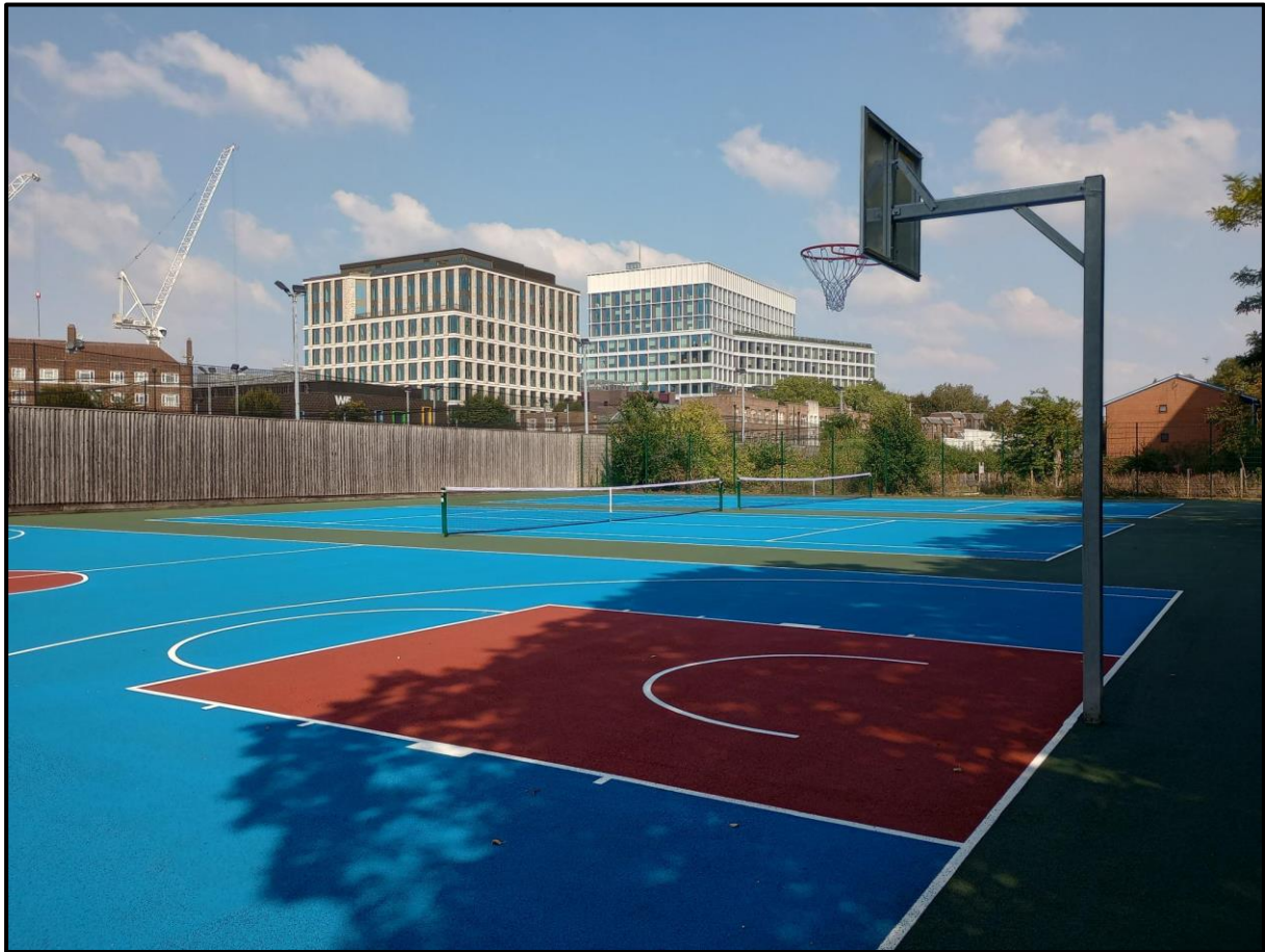
Hammersmith Park's tennis and basketball courts were refurbished in September 2024.
